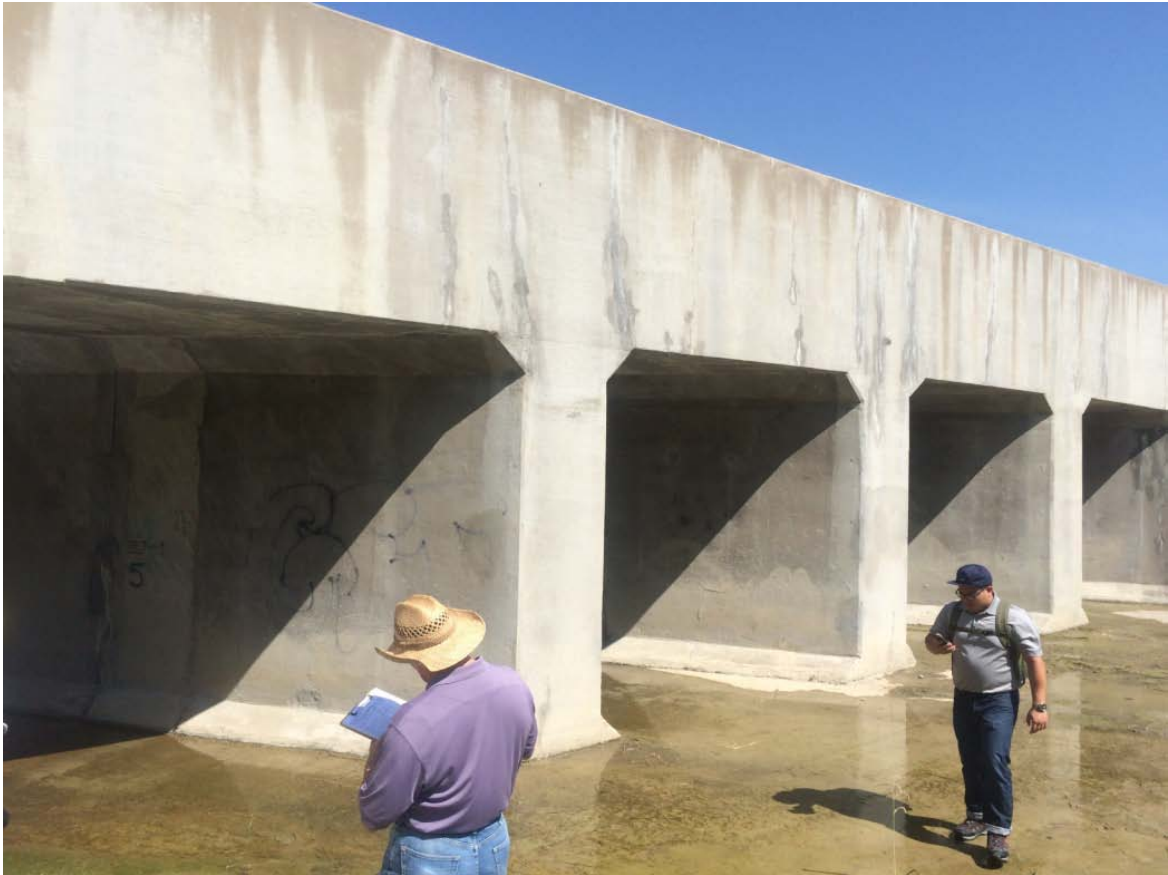
Looking upstream/4 barrel box culvert
