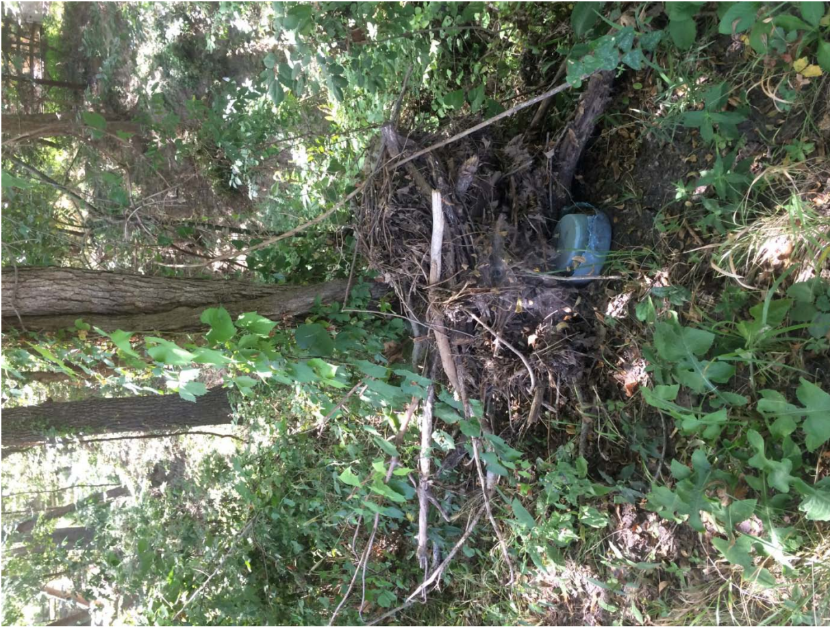
Evidence of stream overtopping the bank
