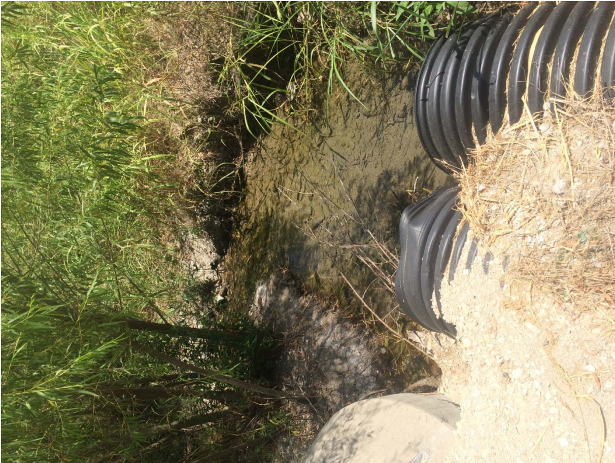
Looking downstream West of 4400.61
