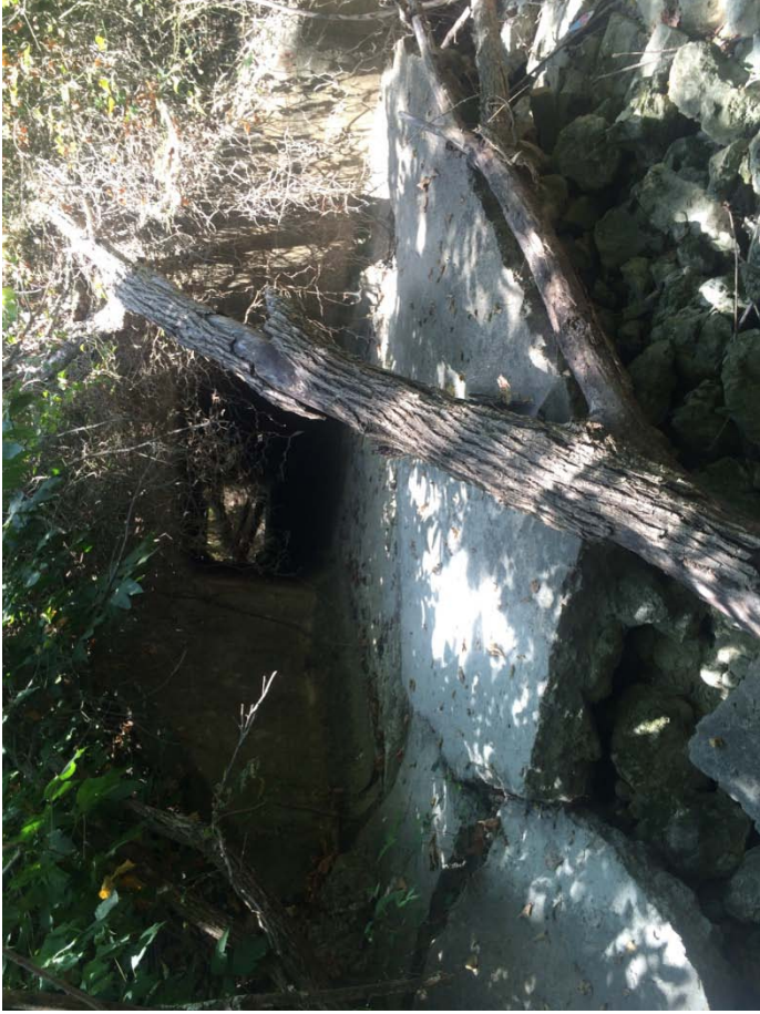
Box culvert running under railroad tracks
