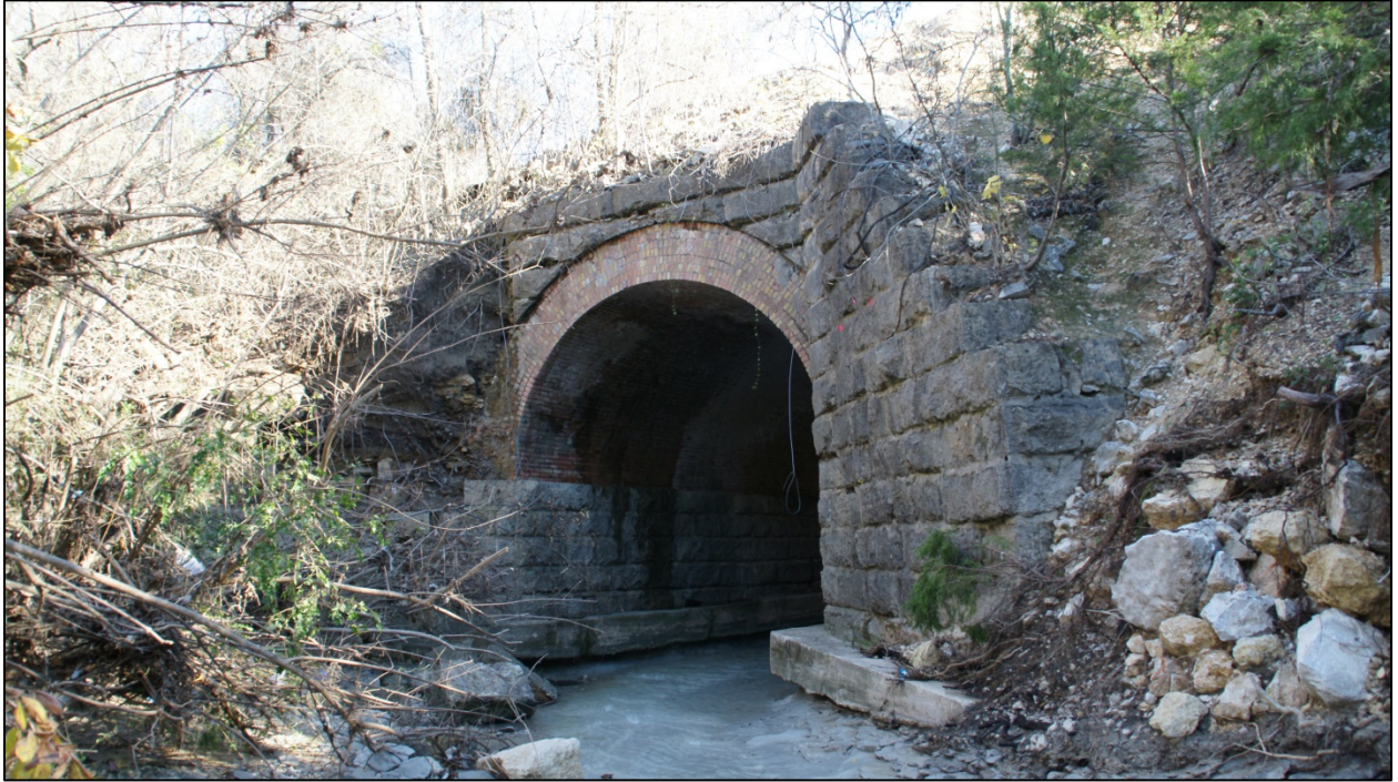
View of Upstream End of Brick Culvert.
