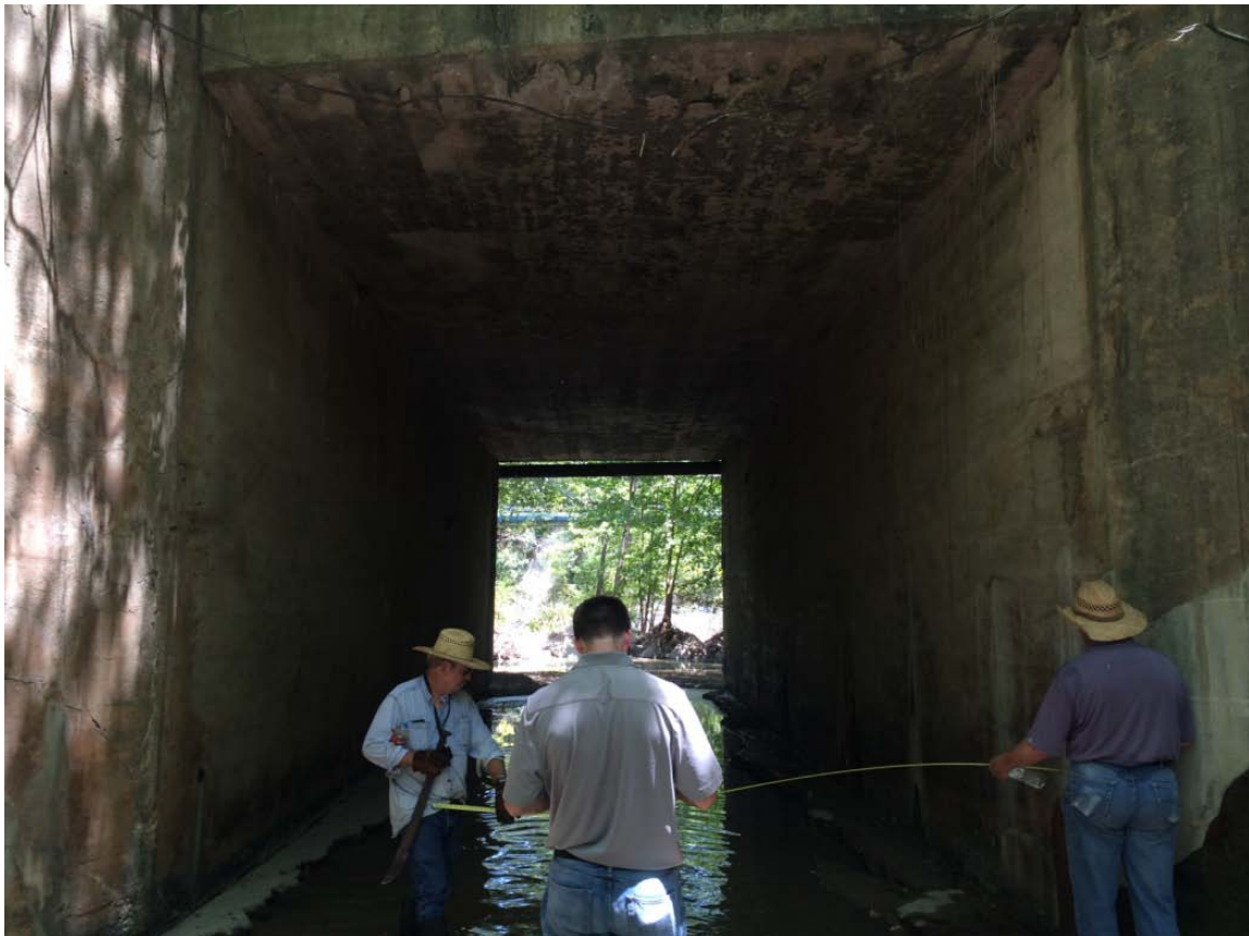
Looking downstream/1 barrel box culvert
