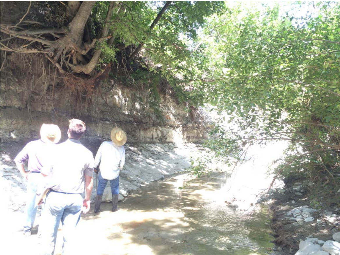
Looking downstream/Left bank
