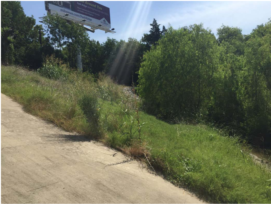
Looking downstream/Left bank
