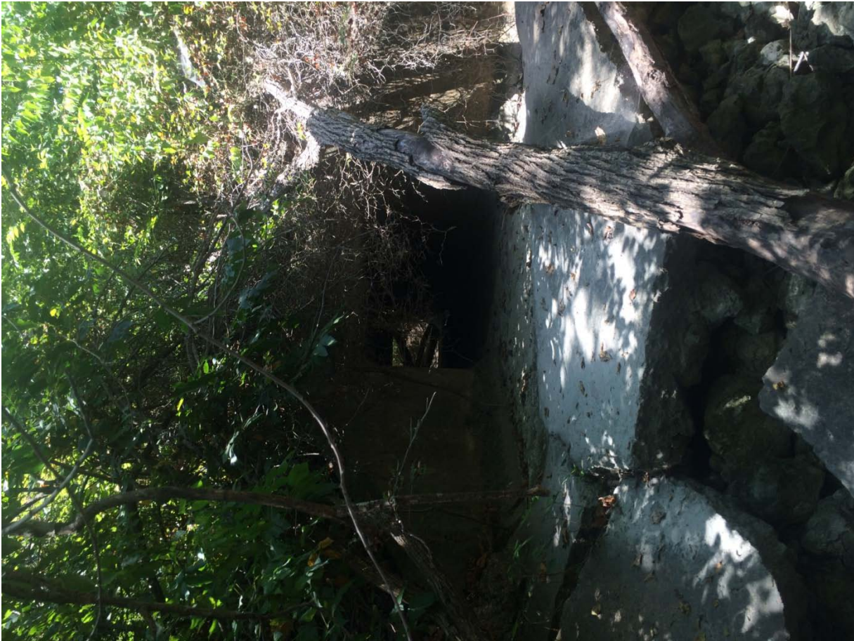
1 of 2 box culverts under the railroad tracks
